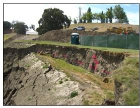
Monitoring involves the maintenance and monitoring of piezometers (measuring ground water elevations), inclinometers, horizontal drains, subdrains, and settlement monitors. Data collected from the instruments is analyzed to establish trends and to attempt to identify slope movement in advance of a landslide or other slope failure.
